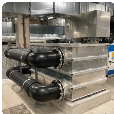
Figure 7: Aluminium StormFilter® tank
