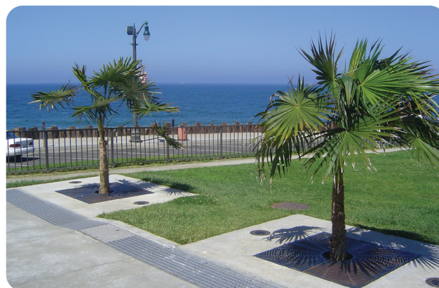
Figure 4: Filterra® tree pit – grated drain inlet
