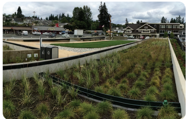
Figure 7: Filterra® bioscape – hard edging
