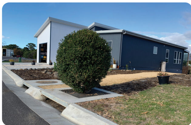
Figure 3: Filterra® tree pit – kerb inlet
