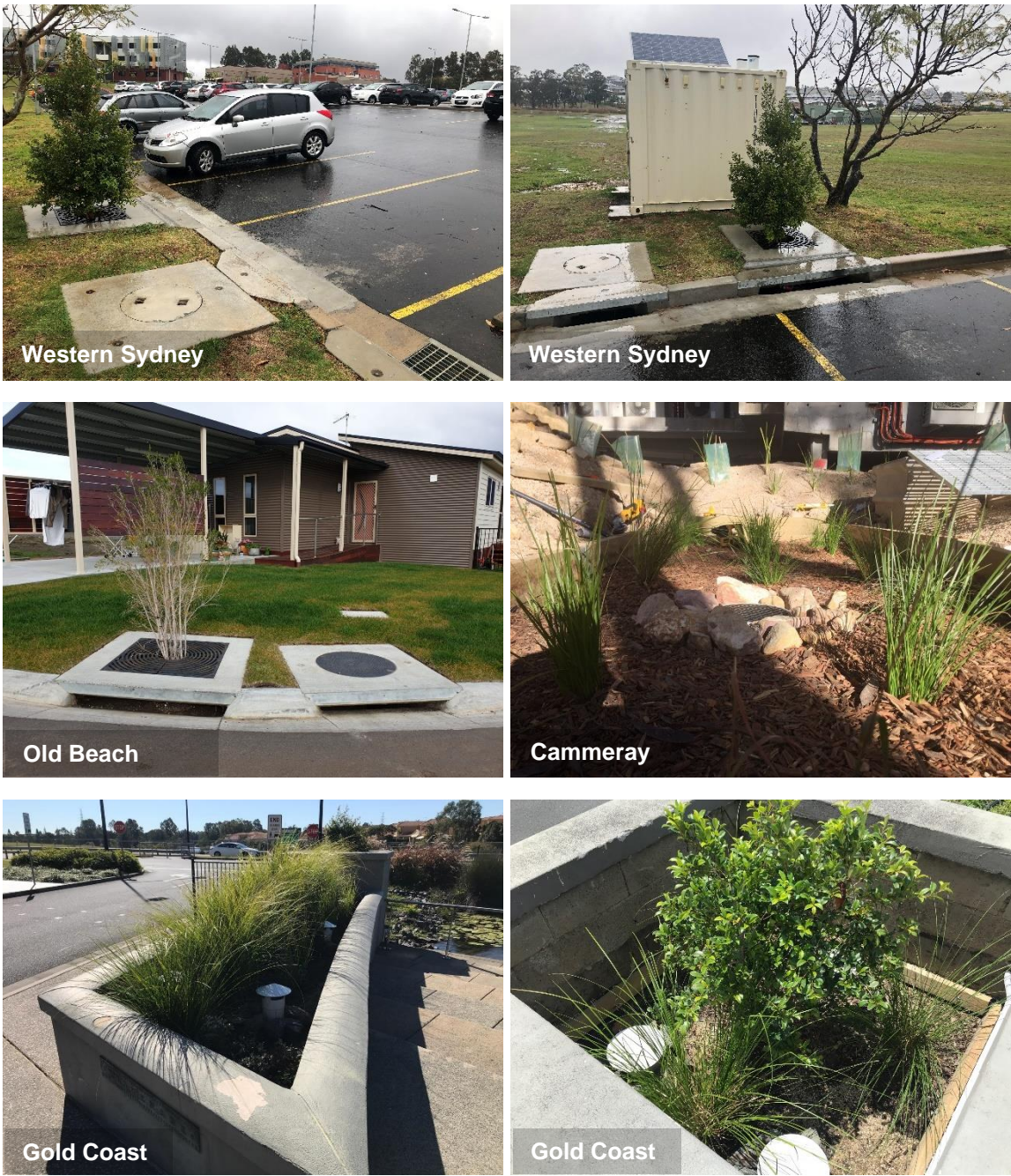
Figure 2-3 Example photos of Filterra® biofiltration systems at Western Sydney, Old Beach, Cammeray and Gold Coast
