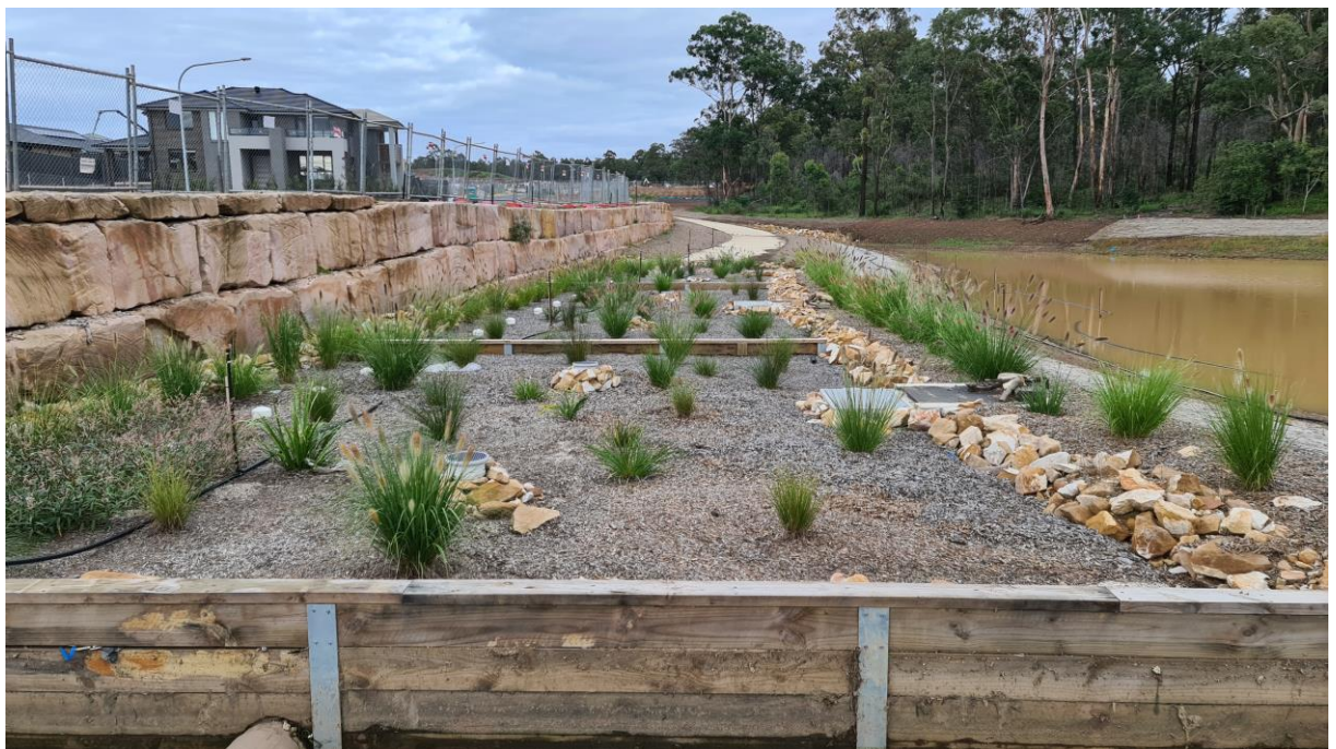
Figure 2-2 Example photos of Filterra® biofiltration systems at Silverdale (during plant establishment)
