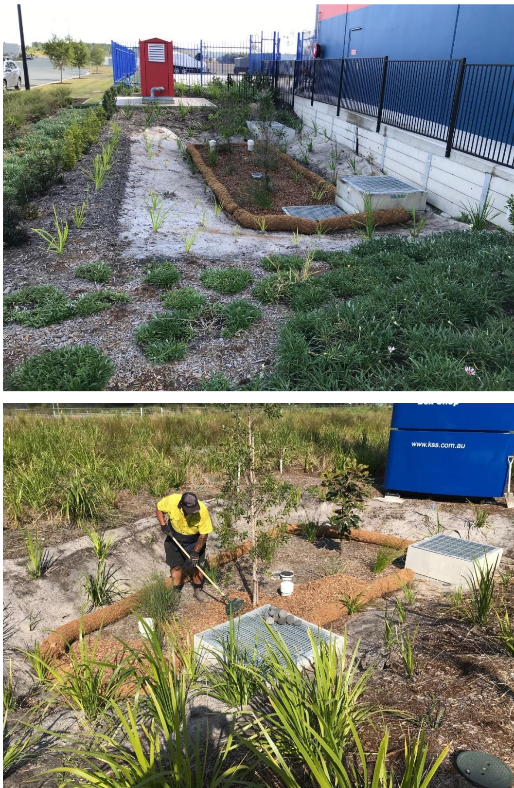
Figure 2-4 Example photos of Filterra® biofiltration systems at Bells Creek (during plant establishment)
