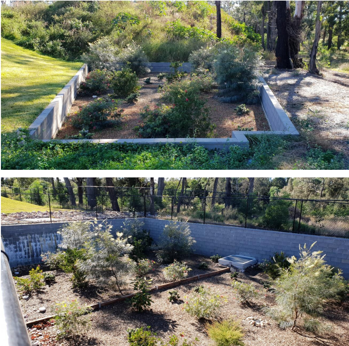
Figure 2-1 Example photos of Filtterra® biofiltration systems at Warwick Farm
