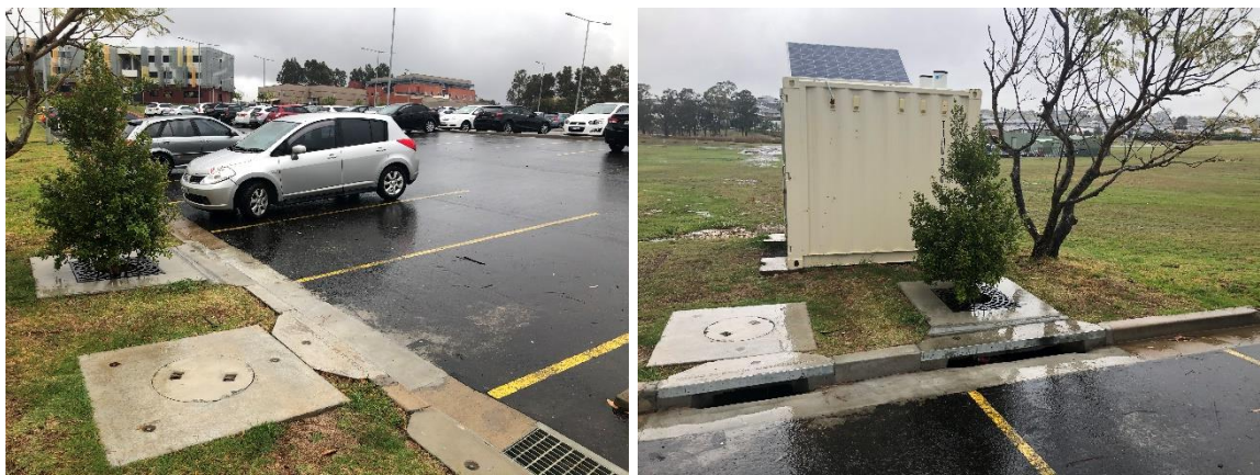
Figure B-3 Example photos of the Filtterra® biofiltration system and sampling facilities at the site
