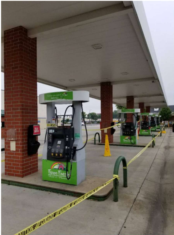
Figure 72. Study site C decommissioning
