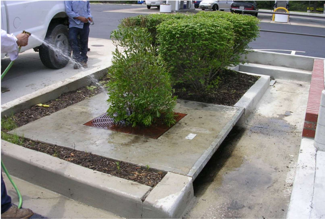
Figure 51. Study site B plant replacement with Northern Bayberry from heavy motor oil contamination in 2005
