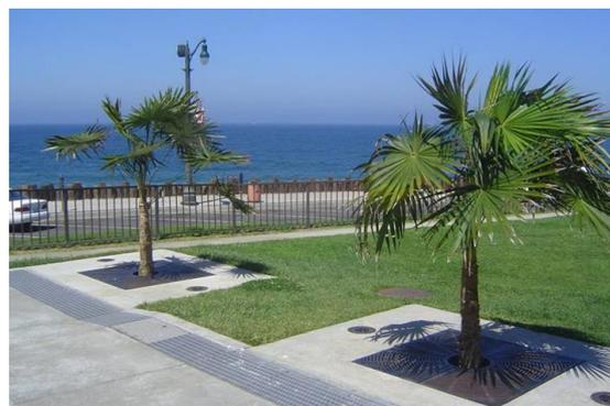
*Figure 4: Filterra tree pit – grated drain inlet*
