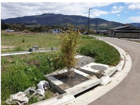
*Figure 3: Filterra tree pit – kerb inlet*
