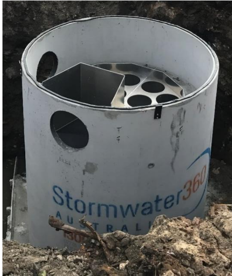
Figure 3: Jellyfish precast manhole
